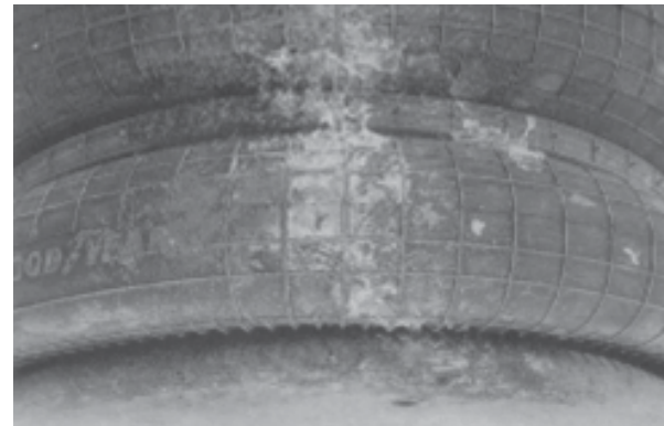
DAMAGE FROM CHEMICALS
